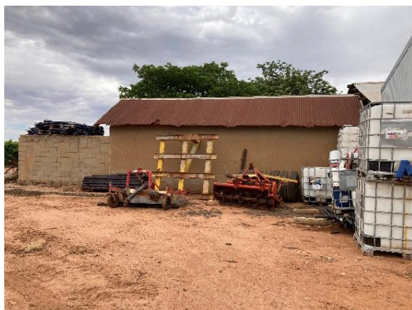
Exterior wall of the cell block.
