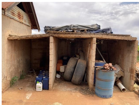
Concrete brick addition to cell block.
