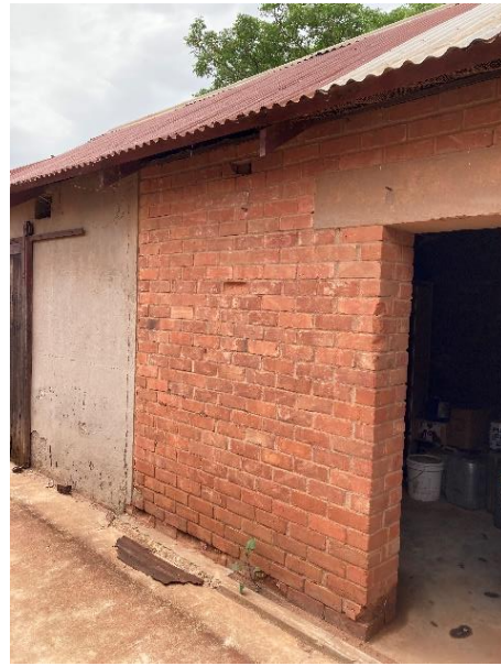
Brick section of the cell block, showing the concrete lintel over opening and channel (now filled with dirt) to accommodate a sliding door.
