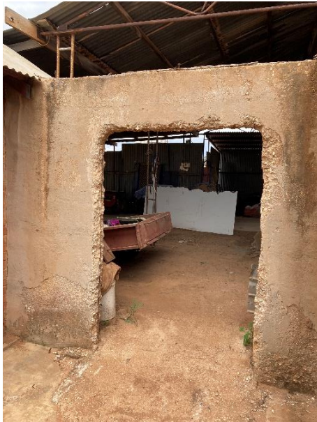
New or enlarged opening in the end wall of the cell block.
