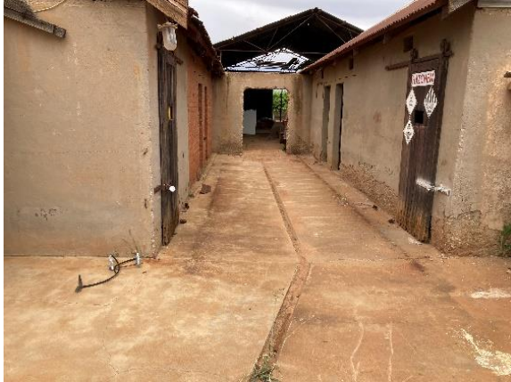
Cell Block showing the cells facing the central corridor, note the drain and sliding door.
