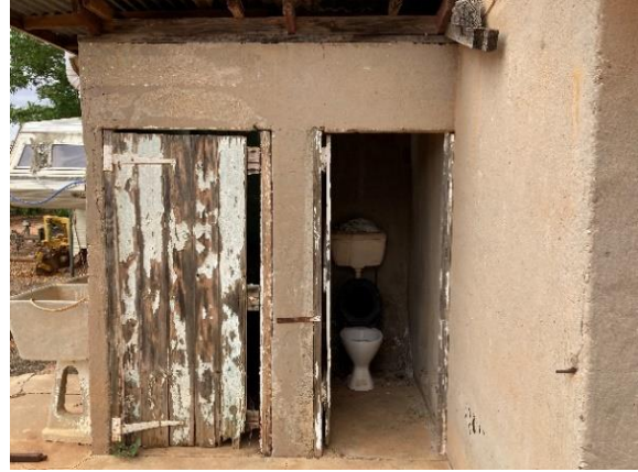
Ablutions block, toilet and shower.
